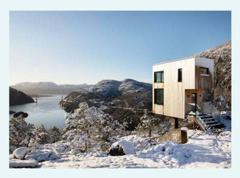
The Bolder Sky Lodges are throned on a single steel column to minimize the landscape footprint. The twinlevel cubes, wrapped in cedar wood, with floor-to-ceiling glazing provide unparalleled views over Norway's Lysefjord.
